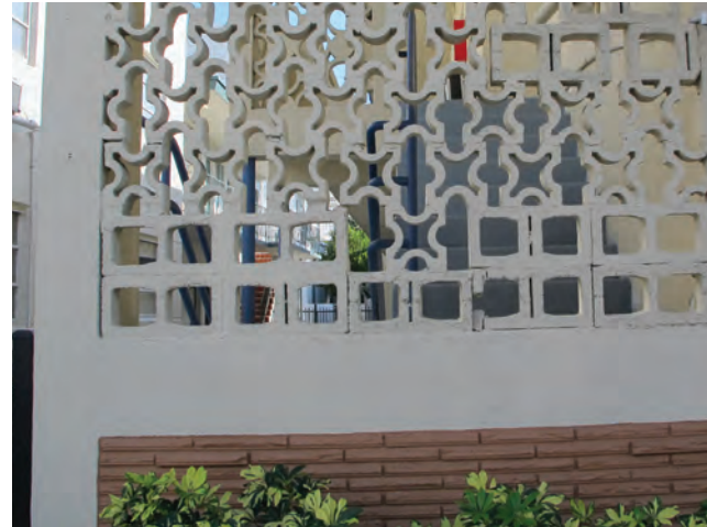
REPAIRS USING INCORRECT MATERIALS
