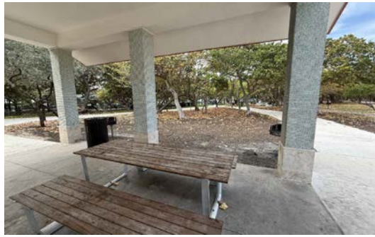
15. BBQ GRILLS, PICNIC TABLE AND TRASH RECEPTACLES - NW VIEW
