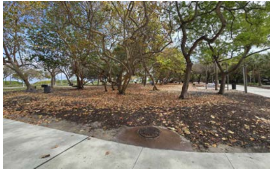
7. BBQ GRILL AND SANITARY MANHOLE - SE VIEW
